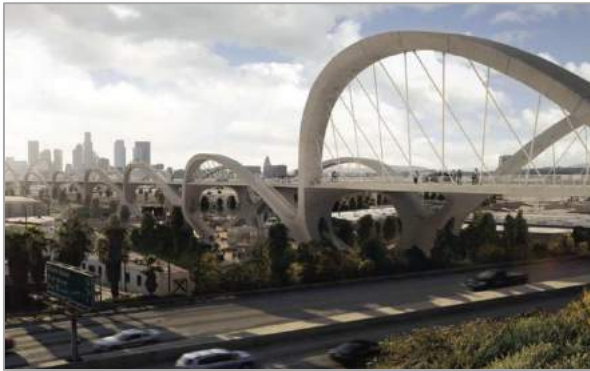
Los Angeles, CA – Sixth Street Viaduct
