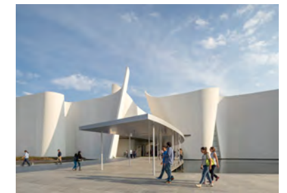
Collective Space and SPECIAL PRIZE Construction Innovation: MIB Cholula, Mexico
